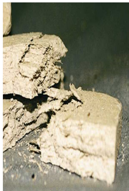
Asbestos insulation board
