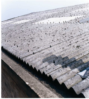
Asbestos cement roof and wall cladding
