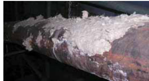
Brown asbestos lagging on in poor condition on steam pipe
