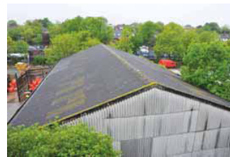
Asbestos cement
