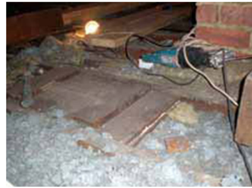
Loose asbestos used as loft insulation
